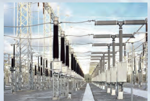
ABB Substation, including transformers and circuit breakers
